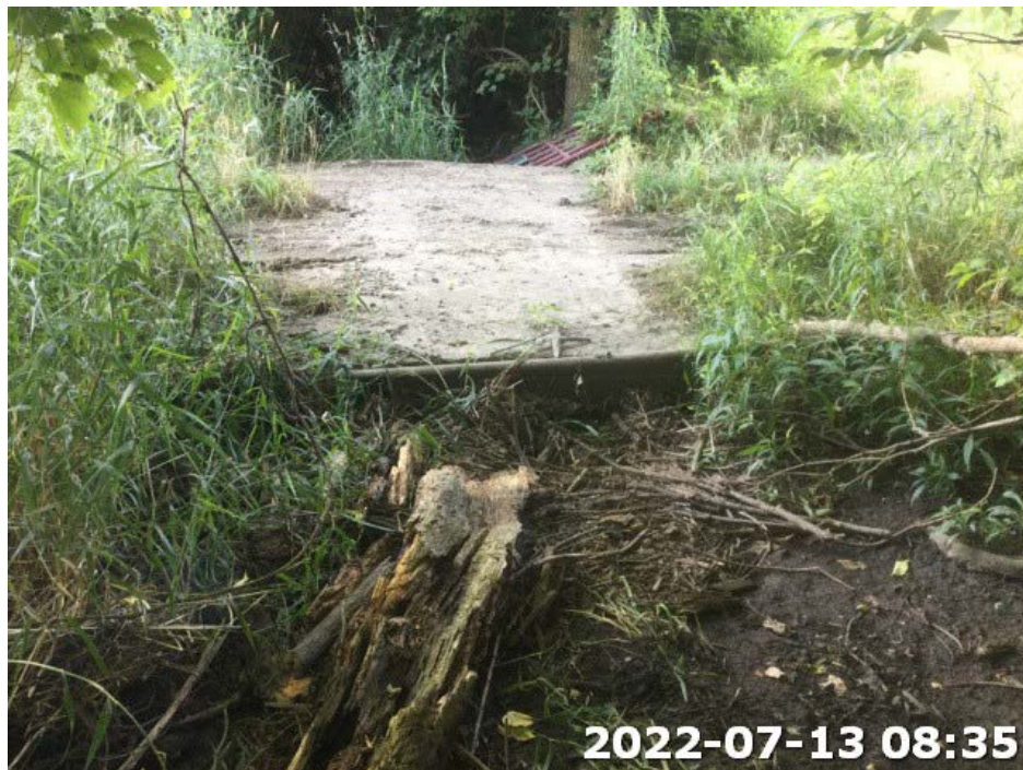
Photograph Location 7. View of existing culvert and upland drainage feature. Photograph taken facing southeast.
