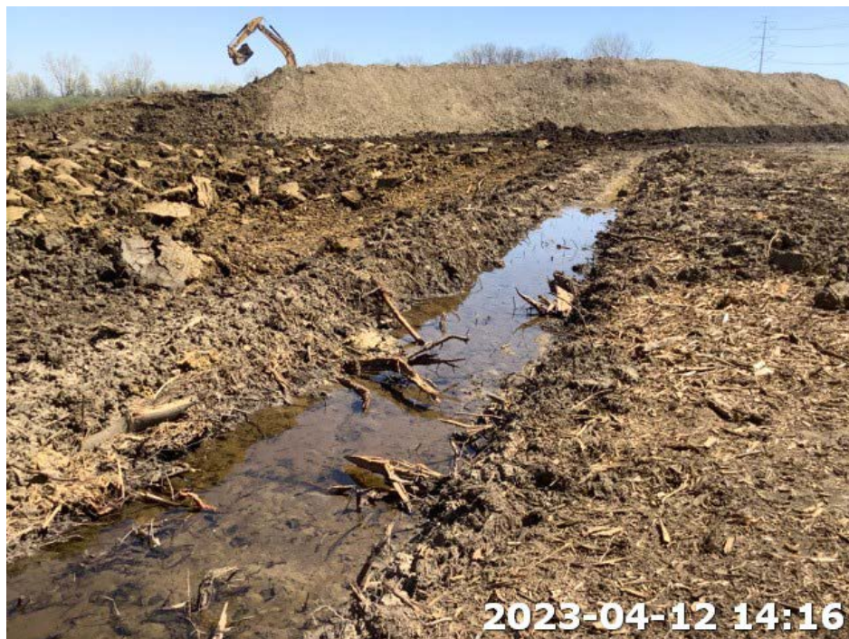
Photograph Location 19. Representative view of upland drainage feature. Photograph taken facing east.
